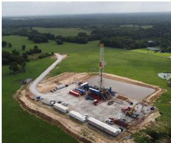
ETX New Well #2 in East Texas.
