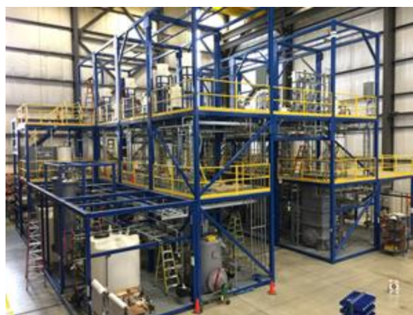
Phase 1 & 2 Modules – photograph taken May 29th, 2019
